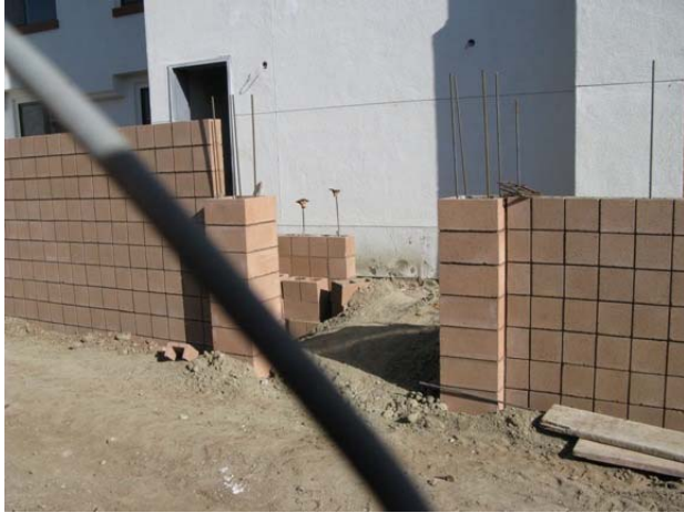
Fig. 1) One of three emergency exits to LWV
